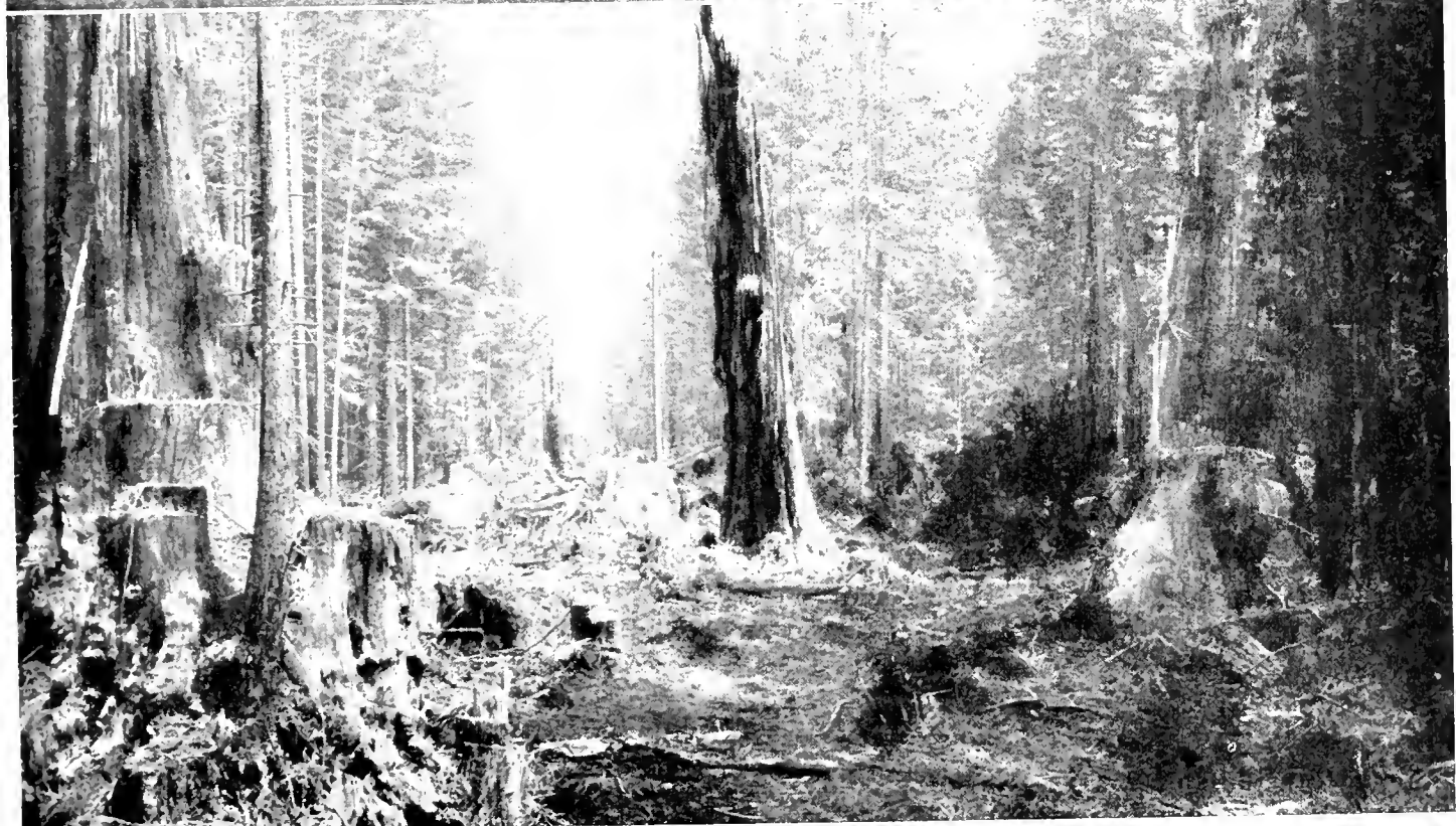
UPPER: This blasting scene has been repeated many times in order to remove the legion of stumps resulting from logging and clearing operations. LOWER: View showing clearing partially completed through an area of dense second-growth redwood forest. The large stumps resulted from logging operations in the 1890's. Approximately one-half of the new alignment passes through this type of forest.
